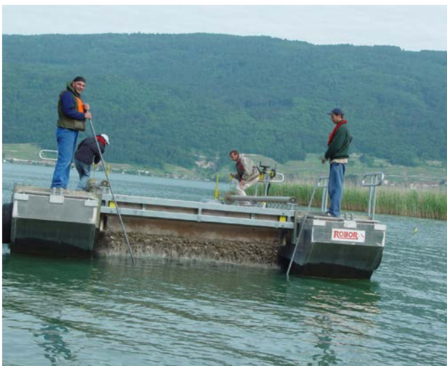
Fig. 5 Dumping of gravel over the laid-out geotextile mats at the site of Sutz-Lattrigen, Hauptstation, Lake Biel. With the help of a special ship equipped with an opening bottom, a thin even layer can be spread, which protects the archaeological cultural layers without creating too much load on them. © Archaeological Service of the Canton of Bern, diving team, 2004.
